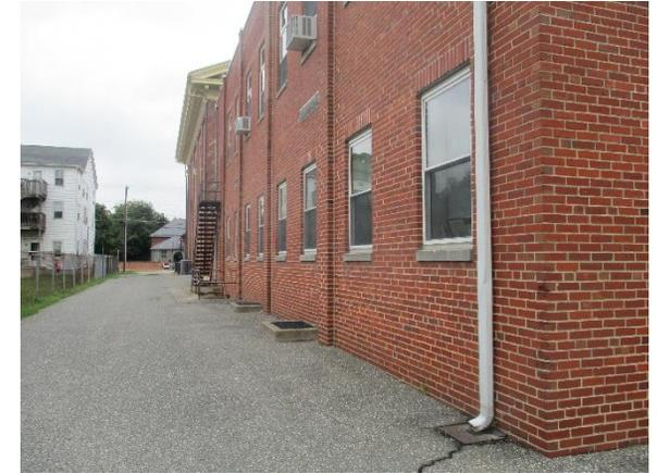
Downspout planter boxes on the east and west sides of the building can capture rainwater from the roof. The harvested rainwater can be utilized to irrigate landscaping as well as reduce stormwater runoff. A preliminary soil assessment suggests that the soils have suitable drainage characteristics for green infrastructure.
