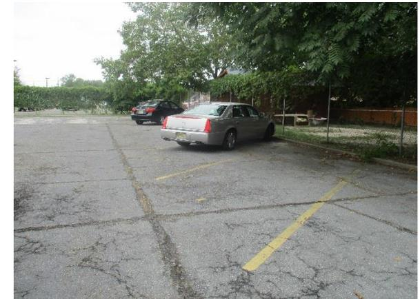
By replacing parking spaces with pervious pavement, the parking lot may capture rainfall and allow it to be filtered and infiltrated into the ground. A preliminary soil assessment suggests that the soils have suitable drainage characteristics for green infrastructure.
